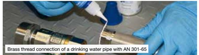
Brass thread connection of a drinking water pipe with AN 301-65
